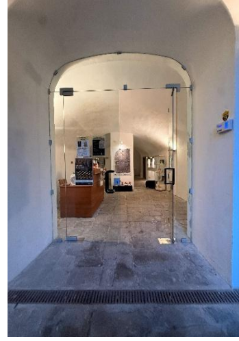
20 entrance with ramp
