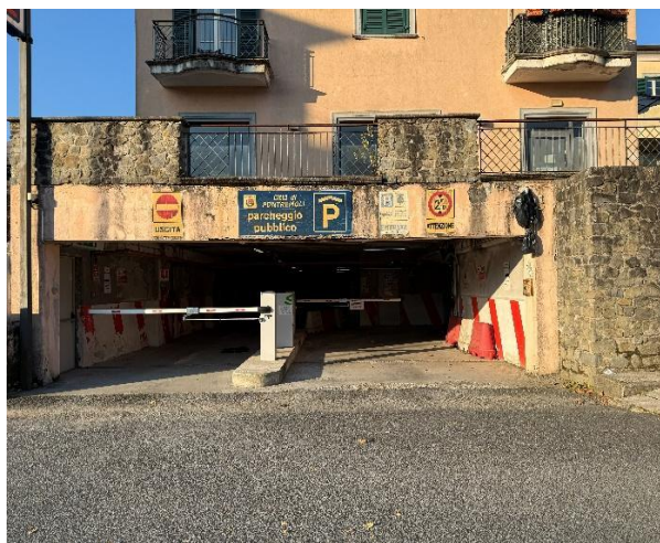
7 Entrance to covered parking
